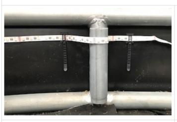
You will need to position a fixing clip either side of each frame section so that the LED strip is secured around the steel upright section.
